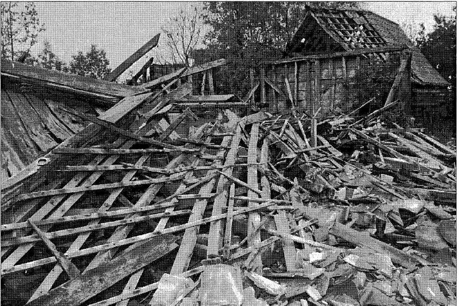
Fig. 1 A barn in Keeley Lane, Wootton, almost completely demolished by the T3 strength tornado of 17th May 1997 Photo courtesy of Times & Citizen
